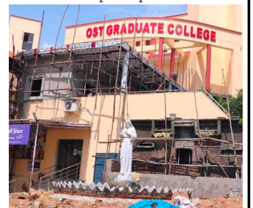
Renovation work in Progress
